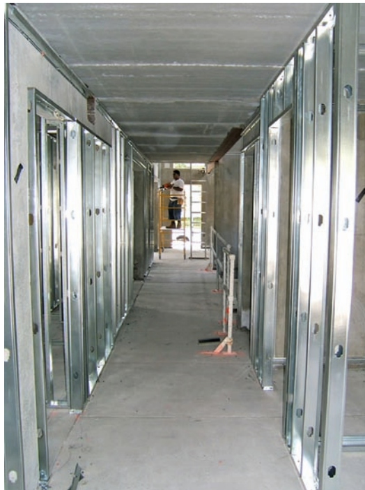
Steel framing was used for faster installation into concrete exterior, floors, and ceilings.
