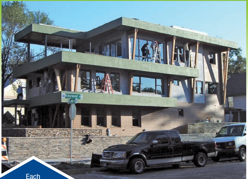
Fiber cement siding and stucco add warmth to the bungalow's exterior.
