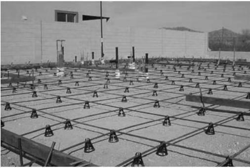
Unbonded monostrand tendons have been used since the 1960's to reinforce the foundations of single and multi family homes, and are now used to reinforce hundreds of thousands of residential foundations throughout the United States each year. This use results in stiffer foundations that protect the house from structural damage due to soils that shrink and swell.
