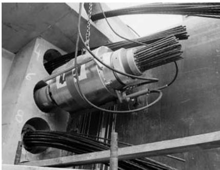
The hydraulic jacks used to tension the post-tensioning tendons range from compact 60 lb jacks used to stress monostrand tendons and small bar tendons, to very large jacks requiring special hoisting equipment, used to simultaneously tension all of the strands in large multi-strand tendons.
