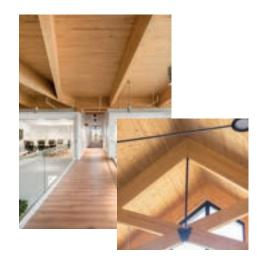
\* This decking alone cannot be used as a diaphragm. Plywood must be added to act as the diaphragm.
