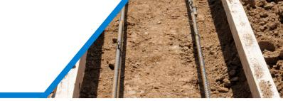
Spacer Bars Ensure A Proper Footing Width When Using Plastic Form-A-Drain® Footings.
