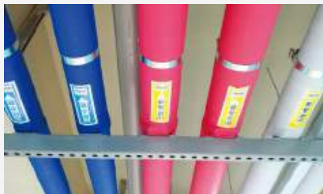
Insulation constructed with magic tape for PIPE
