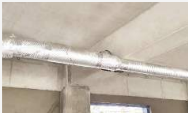
Aluminum foil insulation for PIPE
