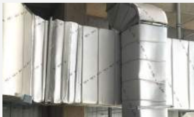
Aluminum foil insulation for DUCT
