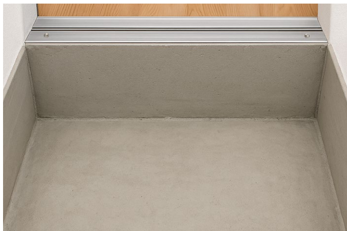
Typical Elevator Pit before Elevator Installation
