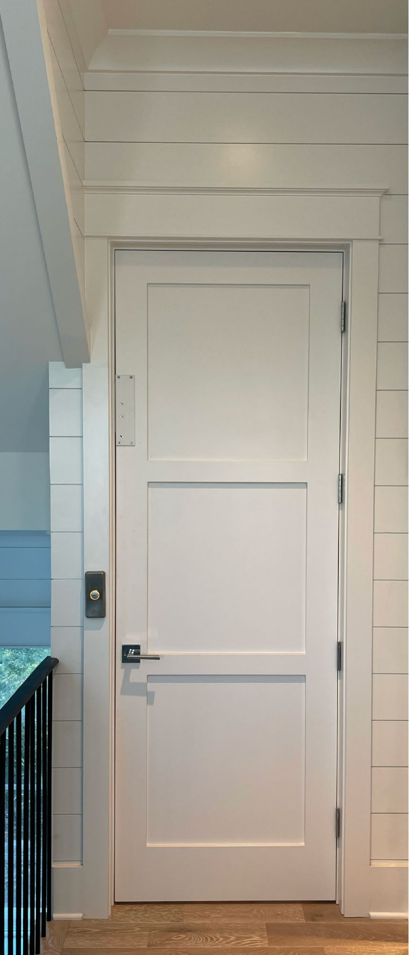
Hoistway Door with Standard Interlock
