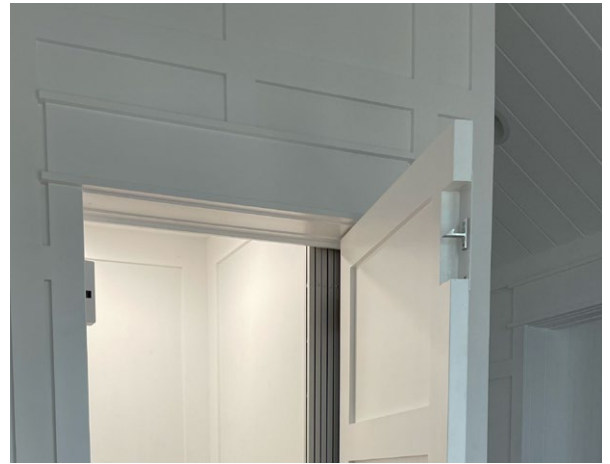
Standard Interlock Installed on Hoistway Door
