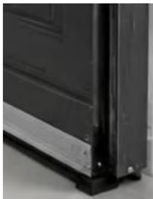
Bottom Weather Seal
