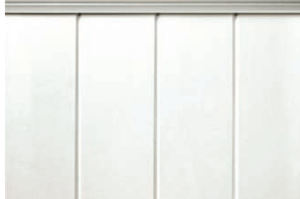
Shiplap WORS6 (smooth side out, 3/16" gap)
