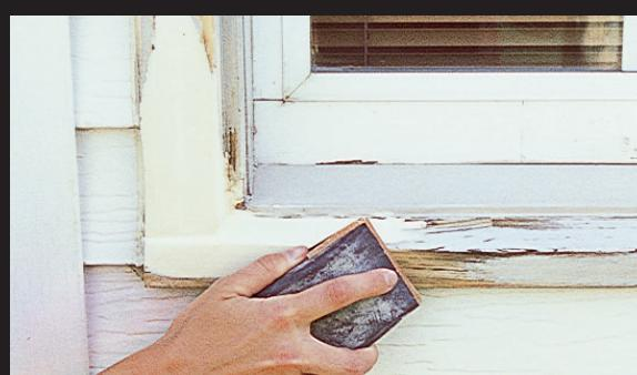
To rebuild missing pieces of wood and fill cracks and holes, apply WoodEpox. When hard, it can be sanded, stained, painted, and nailed.
