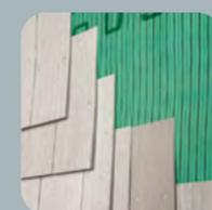
Installs just like traditional cedar shingles. Use exterior grade ring shank (5D Stainless) or siding nails or at least 7/16" wide crown stainless steel staples.
