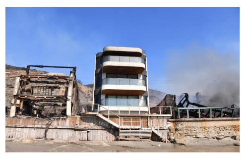
"It's stucco and stone with a fireproof roof," he said, adding that it also includes pilings "like 50 feet into the bedrock" to keep it steady when powerful waves crash into the seawall below it.
