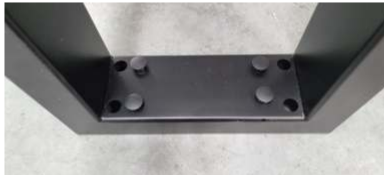
Base of steel frame where dyna bolts Are installed into the concrete floor. Also showing are the plastic covers
