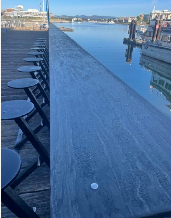
PROJECT: Commercial Restaurant Countertop PRODUCT: Accoya Color Grey unfinished, 1-inch x 6-inch width-laminated into 16-inch-wide countertops LOCATION: Victoria, British Columbia, Canada
