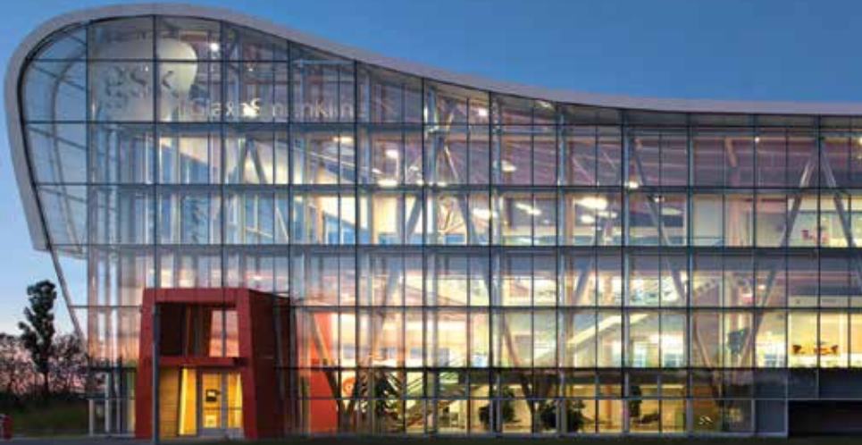
GSK offices. National award: Innovation in architecture
