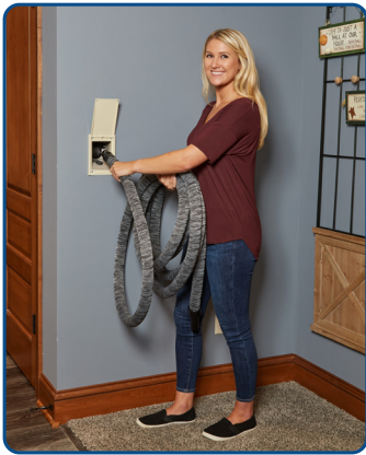
Remove the hose from the Chameleon valve and engage the valve seal.
