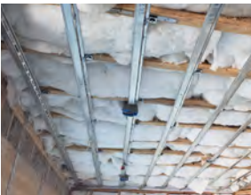
Attachment Slot for RC-1 Channel (screw included)
