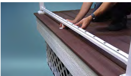
STEP 1: Lay out post locations, leave lags 1" up from baseplate
