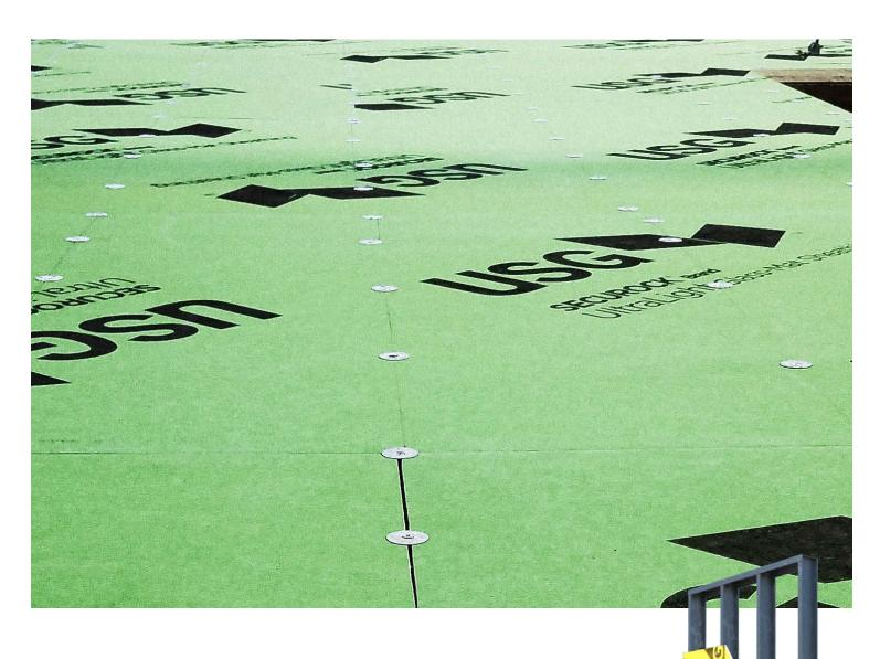
Enhanced mechanical attachment of gypsum sheathing with solid cap steel washers.
