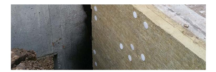
Recommended anchor length 1 1/2"-2" longer than total insulation thickness
