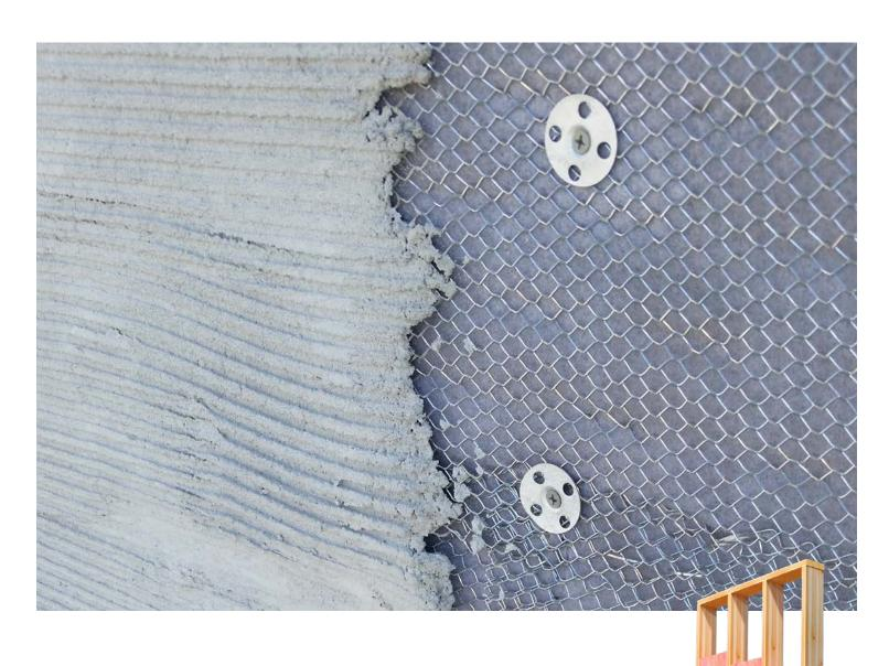
Fasteners to attach insulation and lath for all stucco and lathing:
