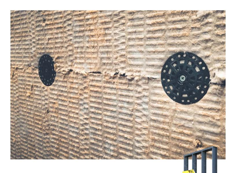
Mechanical attachment of mineral wool insulation.
