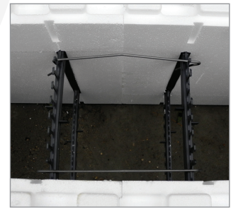
Horizontal Clips in Place
