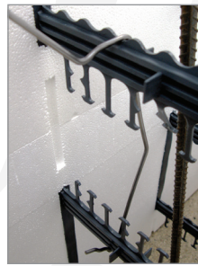
Vertical Clips in Place
