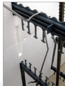
Vertical Clips in Place
