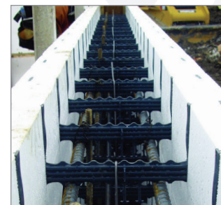
Showing HV Clips holding down a top row that has been cut down to +/- 8" in height
