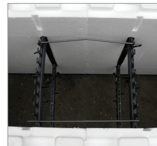
Horizontal Clips in Place
