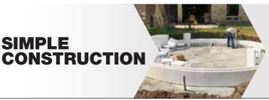
Solid monolithic reinforced concrete provides a high structural capacity for below grade and/or above grade walls, any height, any overall size. Modular ICFs provide a continuously insulated wall with a solid substrate for any pool finish. The base footing and concrete walls must be designed to suit the structural requirements.
