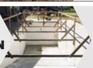
Fox Blocks are 16" x 48" providing 5.33 sq.ft of wall area per block. Installation is very easy and depending on the overall pool layout and design complexity, the blocks for the pool walls and the concrete placement should be able to be installed in one or two days.
