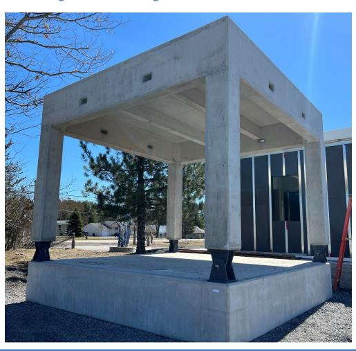
Inserts are cast into the surface of each module, making them ready to receive the next level.
