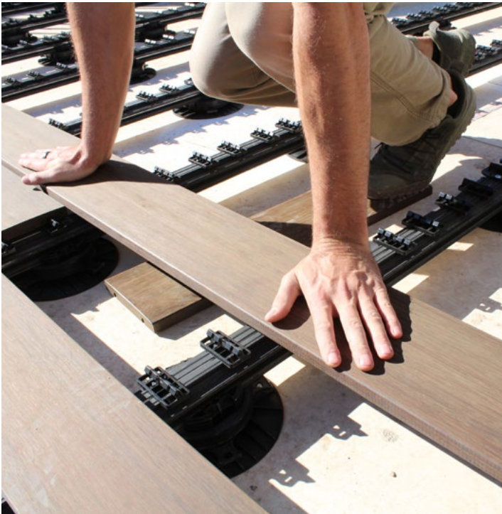
↑ Grad® Decking Installation
